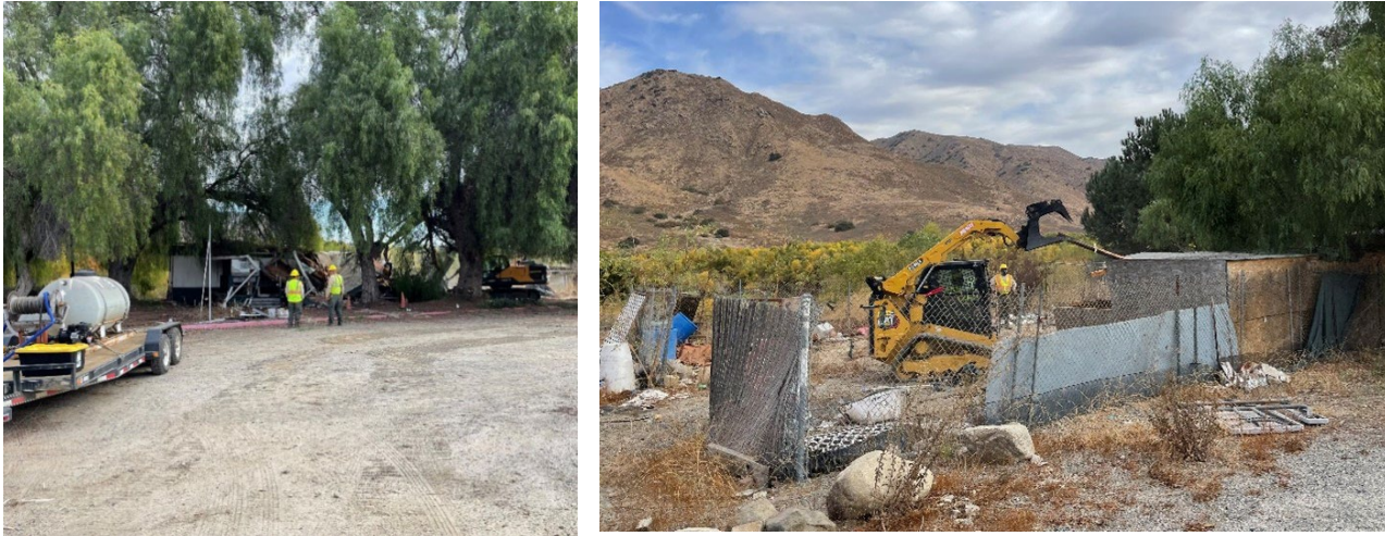
Figure 7-7. Building demolition (left) and cleanup (right) of the Lakeside property.
