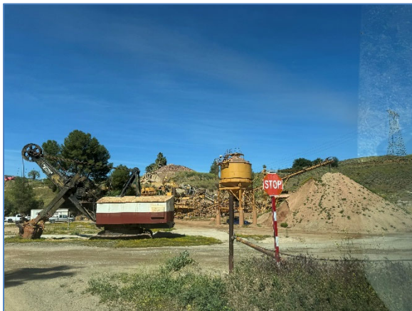
Processing / distribution area
